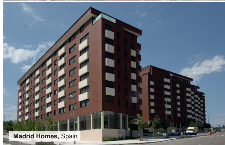
Mostoles Homes, Spain
